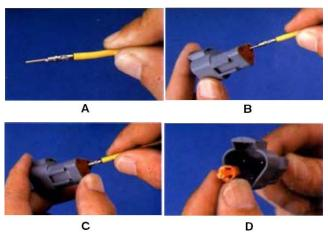
Figure 11-12. DT/DTP Contact Installation
